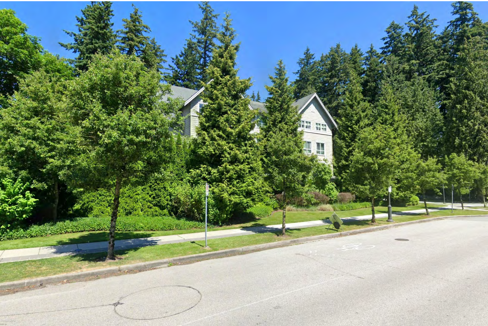
East Campus – TRIUMF House
