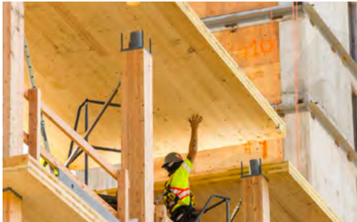
Mass timber construction at Brock Commons Tallwood House. (Photo Credit: KK Law)
